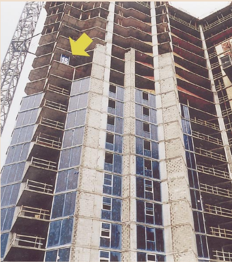
View showing 15th floor from where Mr. Clements fell.
